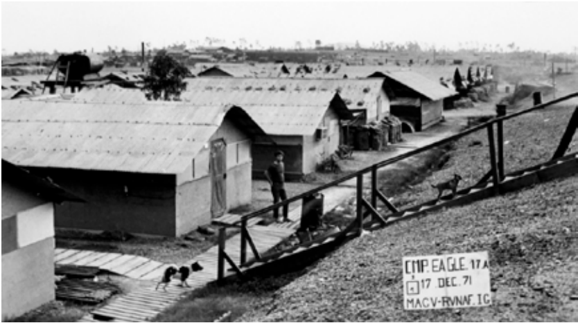
FIGURE 4.5. MACV Base Turnover Files, Camp Eagle. Source: NARA2, RG472, MACV Construction Directorate, Real Property Disposal Files, Box 3. Map software courtesy of ESRI, Inc.
