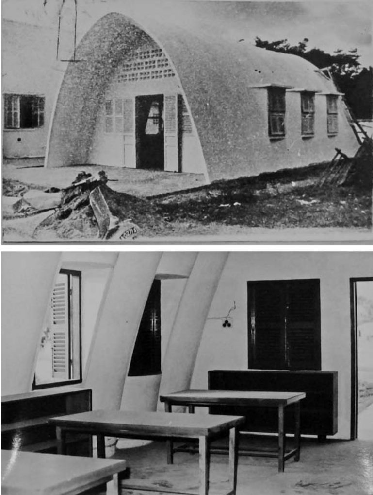
FIGURE 5: High school library made of two conjoined stesiphon huts. Source: "Library 1967," Box 7, Advisory Team 69, NARAC-II.
